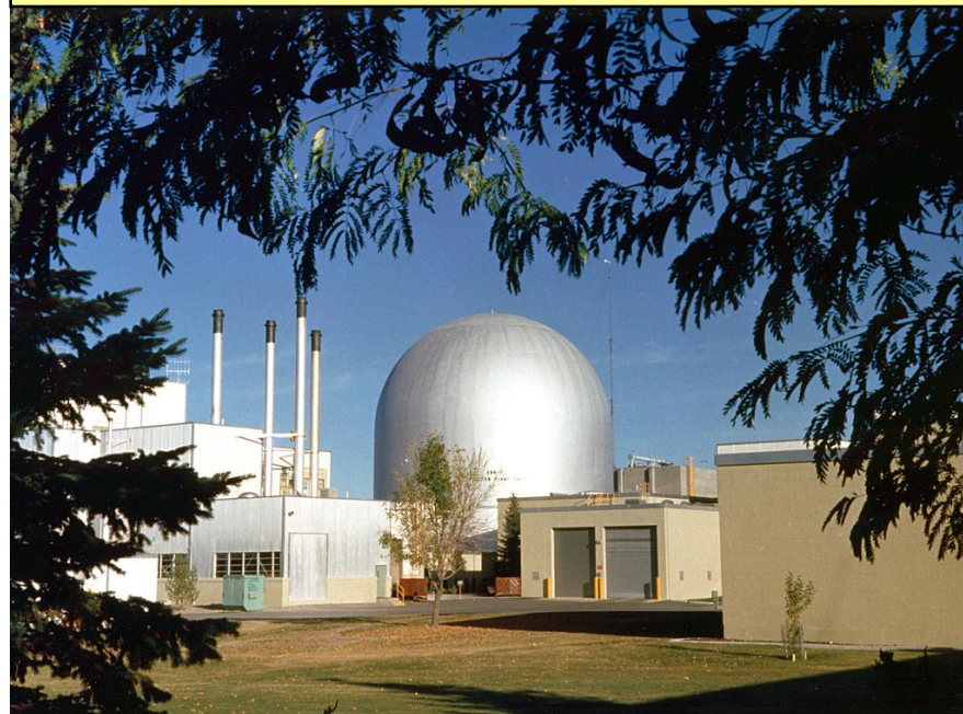
EBR-II sodium-cooled reactor operated for 30 years at Idaho National Laboratory
