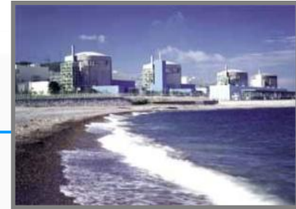
Wolsong Operation - 4 Construction - 2
